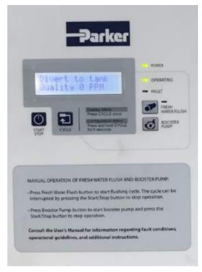
Figure 3.3 – Human-Machine Interface (HMI)/Controller
